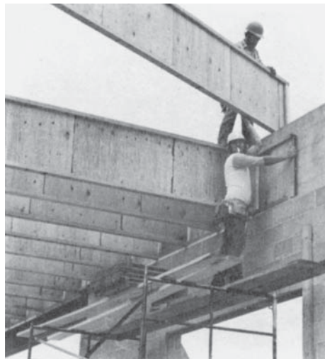
Figure 6.32 c Wood I-joists as part of a wood roof system in a building with masonry walls. (Photo courtesy of Trus Joist—A Weyerhaeuser Company.)
