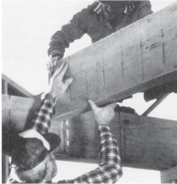
Figure 6.30c Laminated veneer lumber beams. (Photo courtesy of Truss Joist—A Weyerhaeuser Company.)
