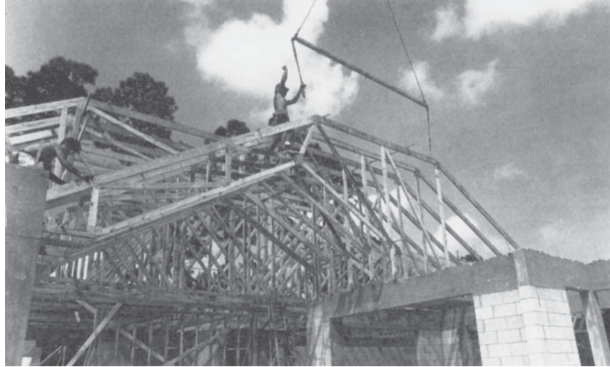
Figure 6.33b Metal plate connected trusses being placed in roof system supported on masonry walls. (Photo courtesy of Alpine Engineered Products, Inc.)
